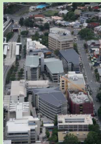
Further progress on the new Southbank Institute of Technology
